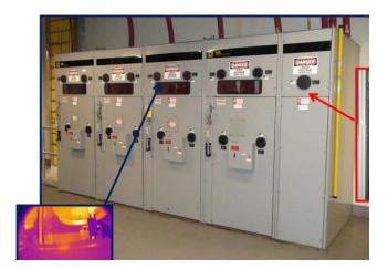
Proper placement of infrared windows is a critical consideration that goes beyond visual aesthetics of the final installation. To maximize effectiveness. window placement must take into account several factors including location of components within enclosures, internal obstacles such as arc barriers, and required field of view. Working with a professional installer or thermographer who is familiar with the subject electrical devices will often yield the best results for window placement.
