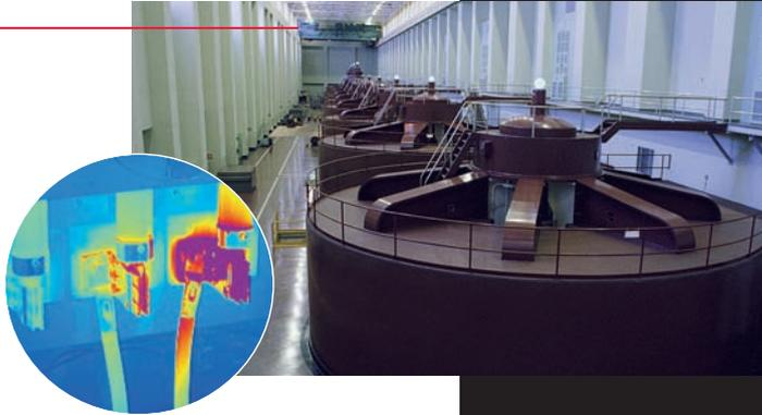
Thermogram shows hot spots caused by defective fuse clips.
